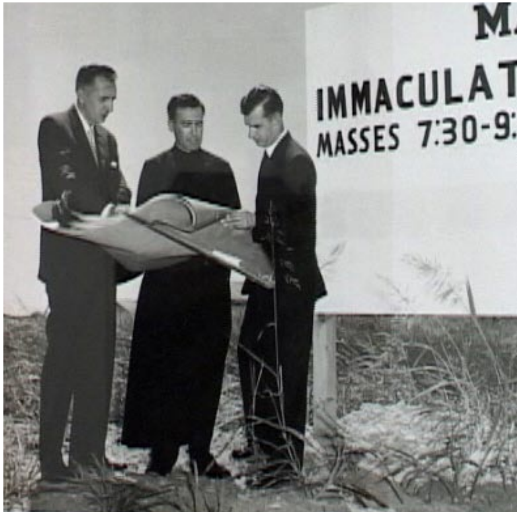
Fr. Robert (center) examining parish blueprints on the land at Valwood and Dennis prior to the groundbreaking for the permanent parish buildings.
